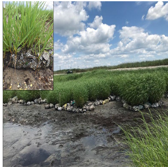
Photo 9: Courtesy of Danielle McCulloch. Photo showing oyster shell bags protecting eroded edges of spartina patches and supporting new growth at Gandys Beach, NJ.
