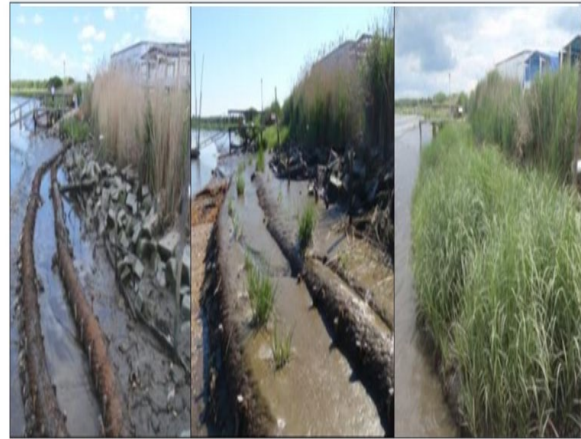
Photo 8: Courtesy of Dr. Josh Moody. Photo showing coir logs stabilizing sediment and supporting vegetation growth at eroded marsh
